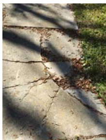
Cracked sidewalk
